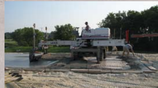
This laser screed is capable of pouring large indoor and outdoor concrete floors
